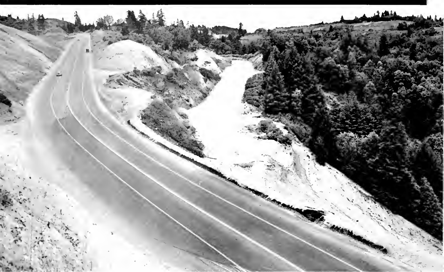
Completed repair of slipout at junction of old and new highways 12 miles north of Santa Cruz. Dark pavement marks area of slipout.
